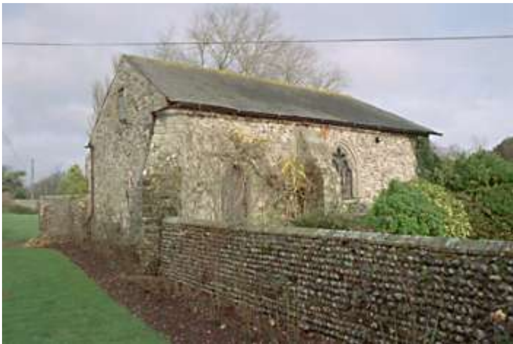
Plate 5: The chapel at Otteham court to the north west of the house.
