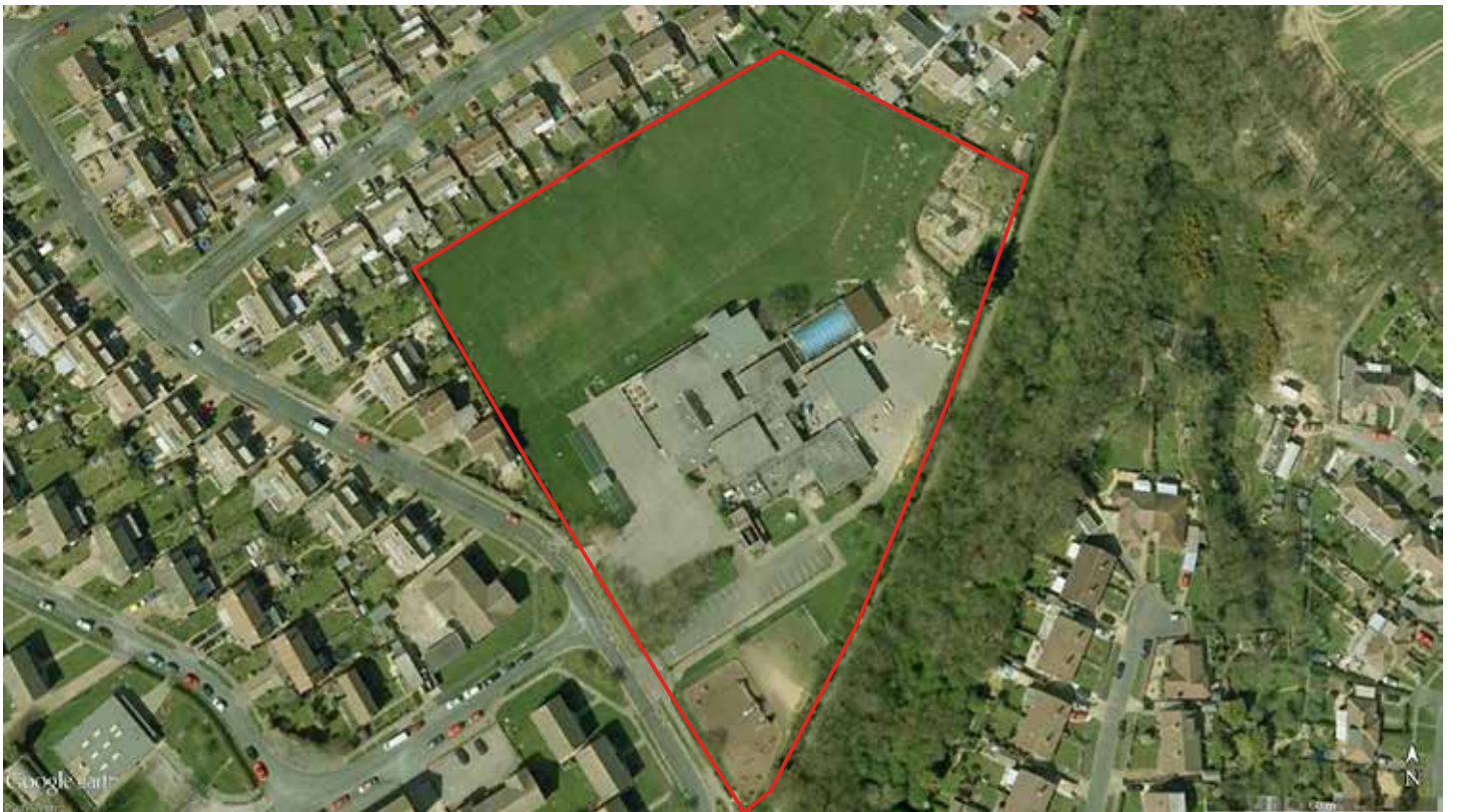
Plate 2: Google Earth aerial photograph from 2006
